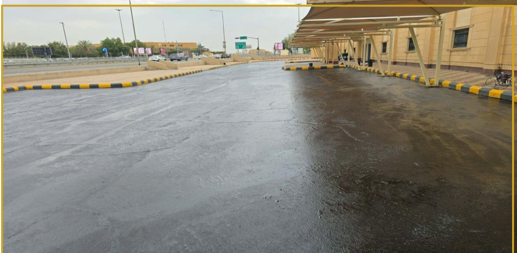
رش الختم الضبابي | Fog seal spray application in progress
